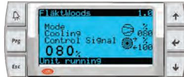
This screen displays information related to the current status (operation mode) of the coils (condensing/evaporating) and whether the AHU is configured with supply air in the upper or lower level.
